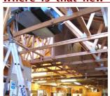
The Clubroom upgrades are well underway, including two air-conditioning units, a fully enclosed attic space and a plastered ceiling.
