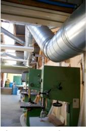
As you would be aware, the Clubrooms have been effectively closed for the past three weeks to allow for the installation of the new dust extraction system. Virtually all of the ducting is in place, and we are only awaiting the arrival of the control system (which is manufactured by a third party), to enable the final wiring to be completed.
