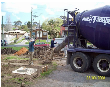
Pouring the Foundations
