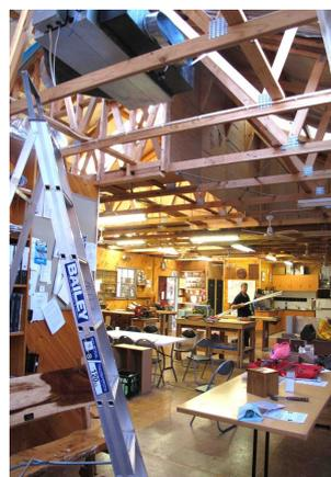
The Clubroom upgrades are well underway, including two air-conditioning units, a fully enclosed attic space and a plastered ceiling.
