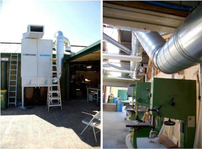
As you would be aware, the Clubrooms have been effectively closed for the past three weeks to allow for the installation of the new dust extraction system. Virtually all of the ducting is in place, and we are only awaiting the arrival of the control system (which is manufactured by a third party), to enable the final wiring to be completed.
